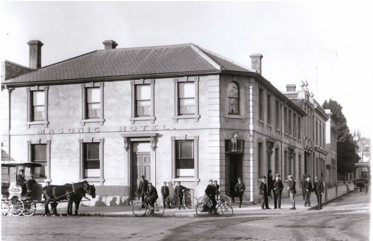
Masonic Hotel 1902 (Note rendering of external walls and trim of windows since 1895 photo)
