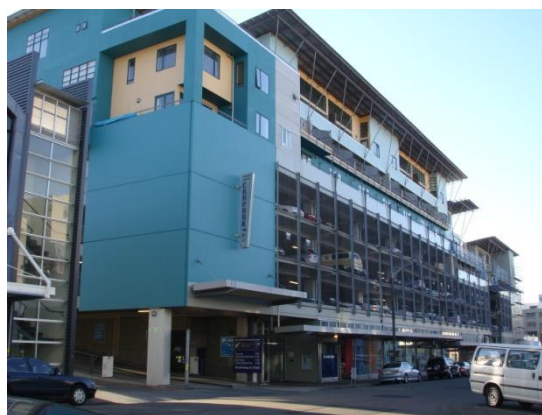
2007 Marion St Car Park & Apartments including 28 Marion St
